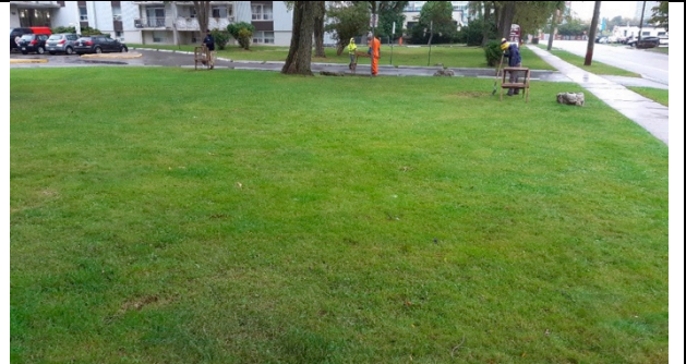
IMAGE 6 TEST PIT SURVEY CONDITIONS (UNDISTURBED GRASS LAWN) AND CREW AT WORK
