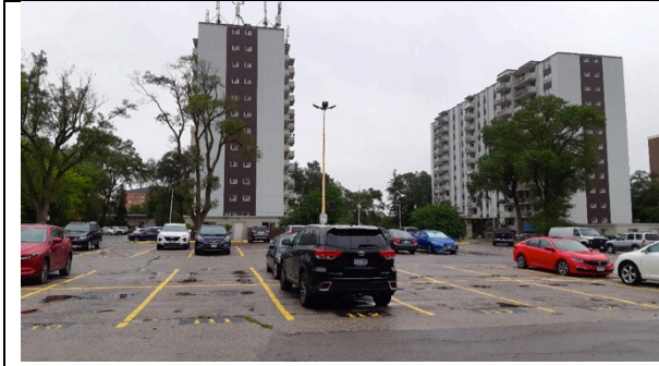
IMAGE 1 2570 & 2590 ARGYLE ROAD APARTMENT BUILDINGS AND PAVED LOT
