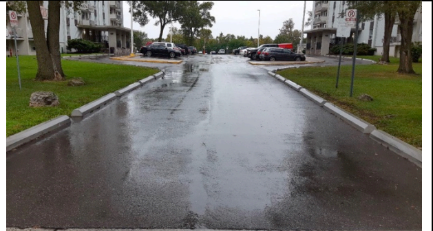
IMAGE 2 PAVED ROAD BETWEEN APARTMENT BUILDINGS
